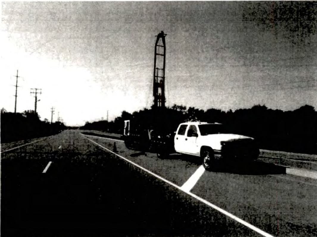
Photo 4: Boring P-2 was located in the center of Veterans Blvd.
